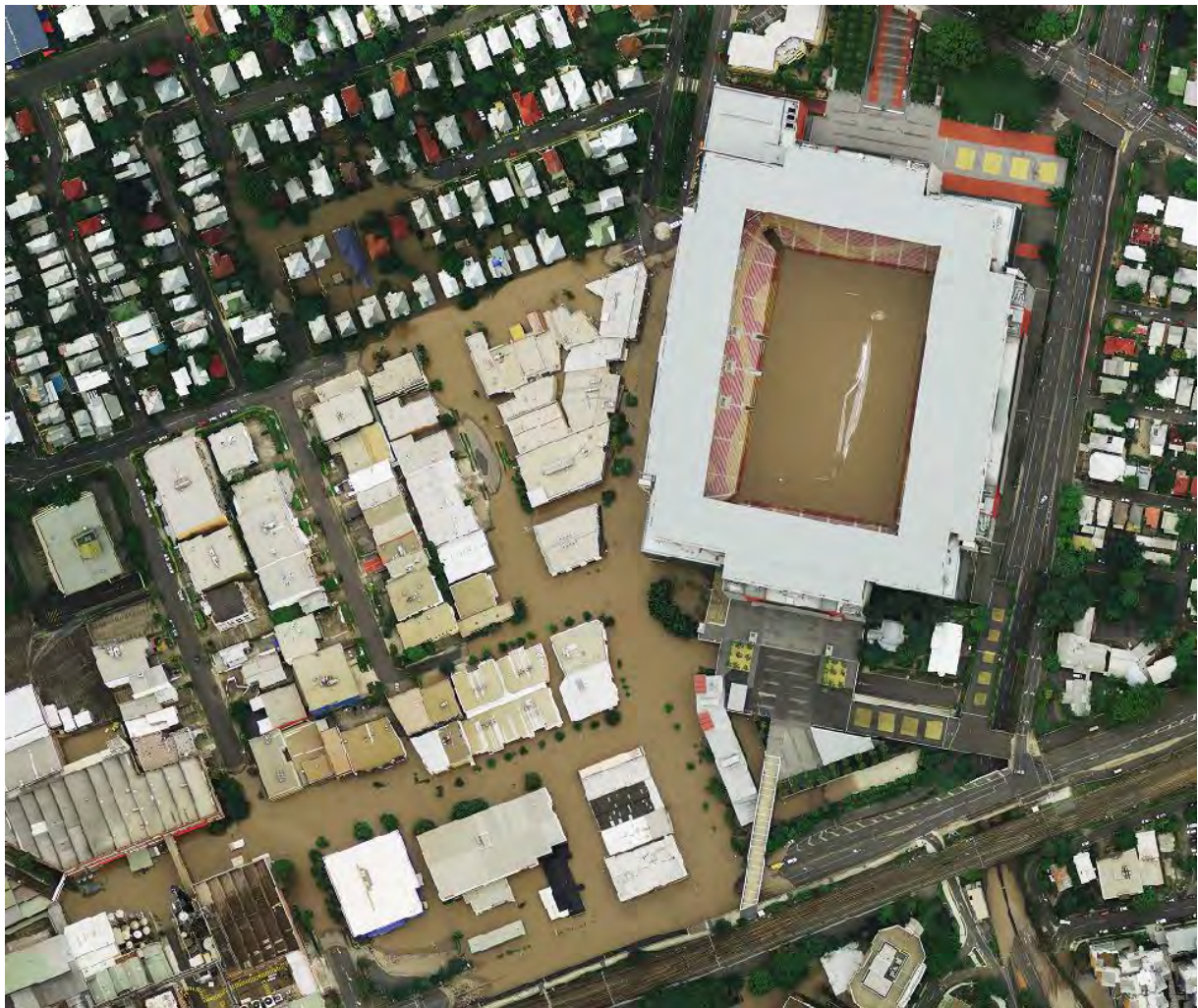
Figure 4-1 Aerial Imagery of the 2011 Flood at Suncorp Stadium
