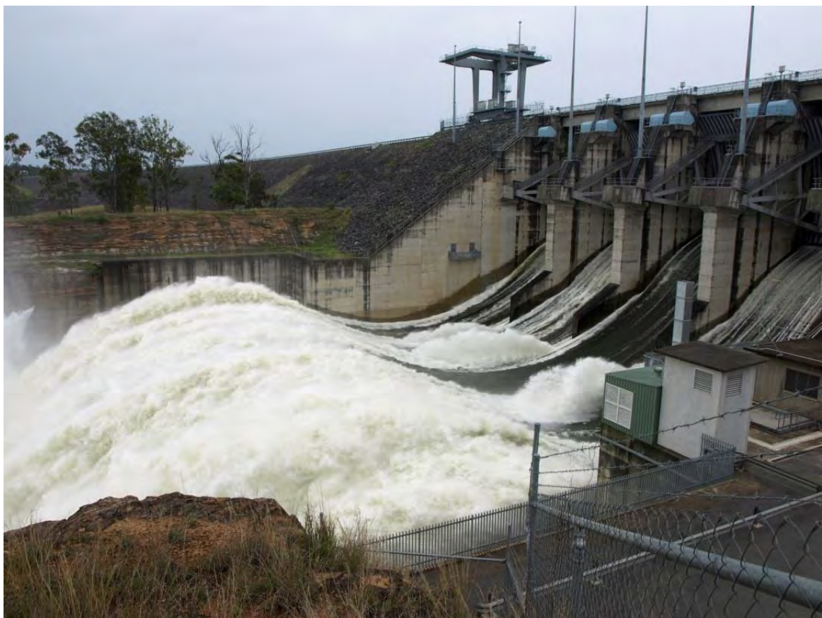
Figure 2-2 Wivenhoe Dam Spillway Releases (October 2010)
