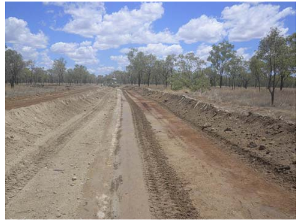
Gregory Developmental Road – preparation work prior to gravel re-sheet
