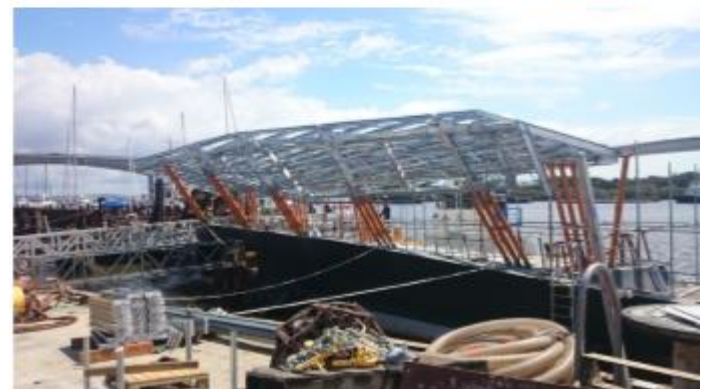
Right: Fit out of gangways (top); and pontoon roofing and ceiling cladding works on the portal frame and over-water waiting area at Regatta terminal (bottom)
