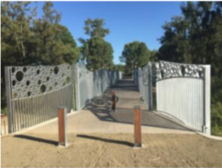
The completed Toogoolawah pedestrian bridge
