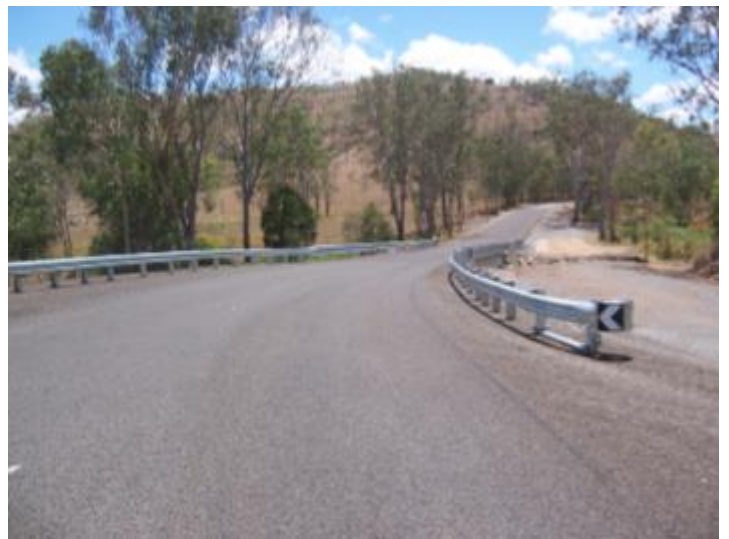
The completed Jones Bridge on Gregors Creek
