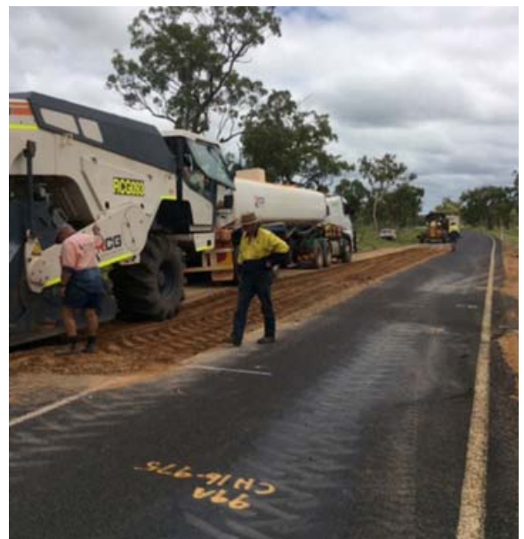
Kennedy Developmental Road – commencing pavement stabilisation
