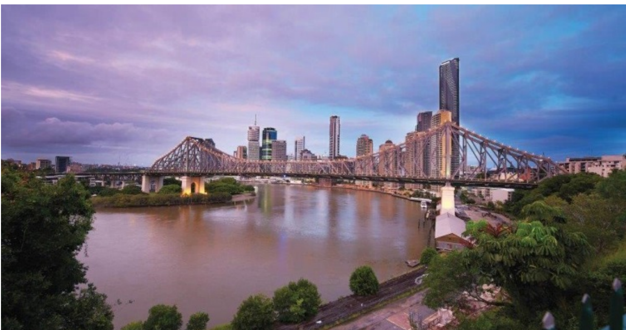
View of the Story Bridge in Brisbane from above the Howard Smith Wharves.
