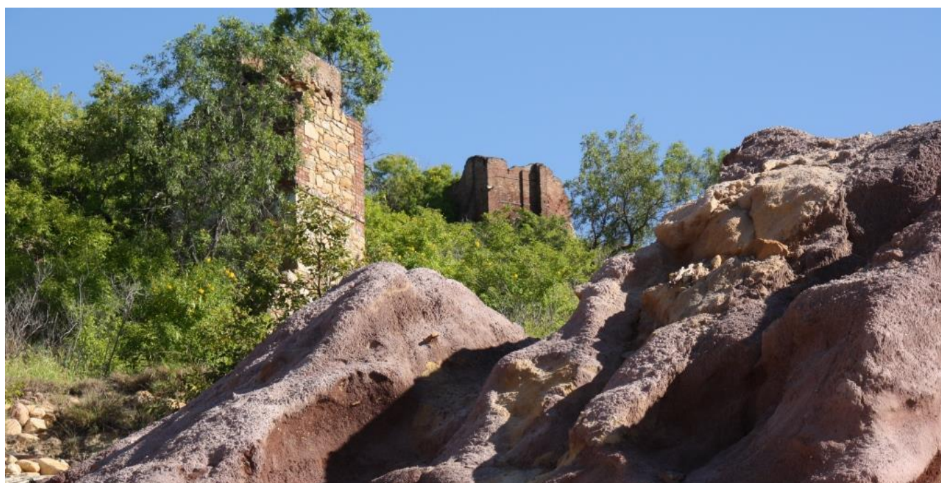
Pyrites Works at Towers Hill in Charters Towers.
