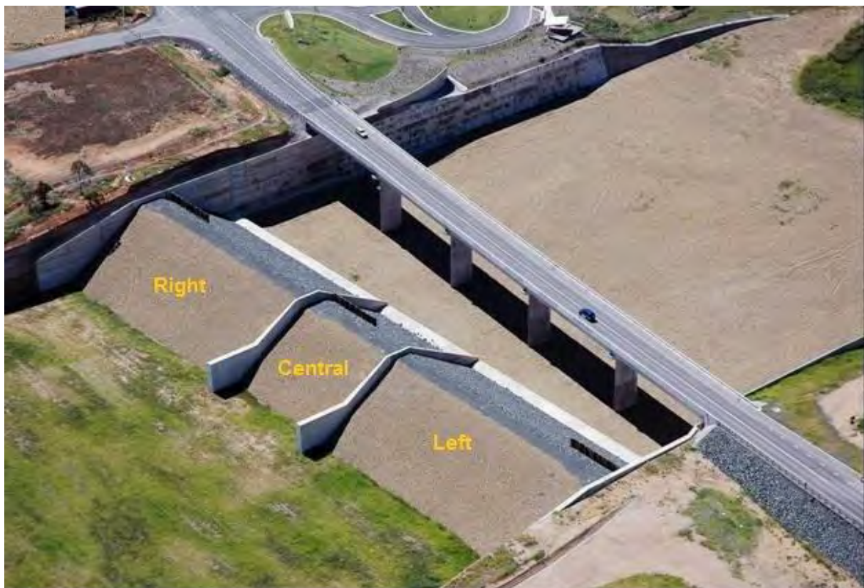
Figure 2.2 Wivenhoe Dam auxiliary spillway and fuse plug bays
