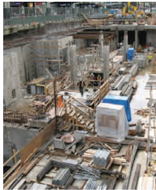
Bottom up construction
