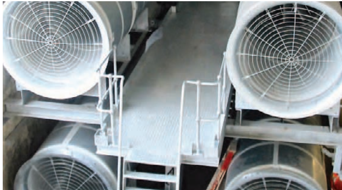
Top: Cross passage between tunnels
